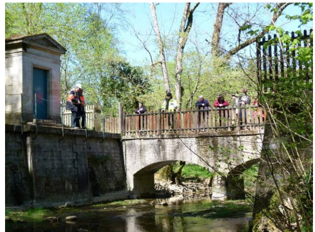
Rosoir Spring in the Suzon valley. The structure on the left is one of a pair of access points to reservoirs which capture the spring water.
